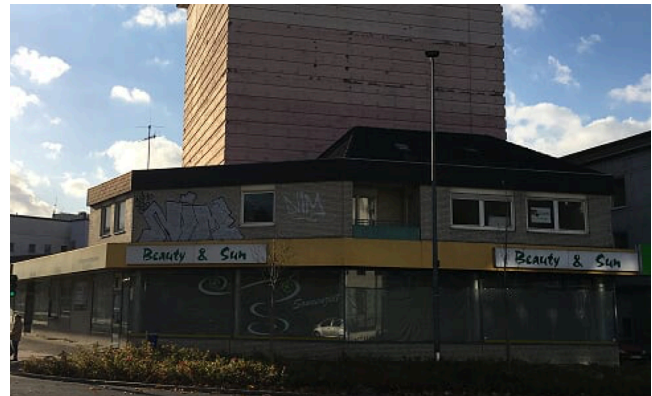
Figure 3: The spatial proximity between the sign of the shop (bottom) high-rise bunker (above) is too low.
